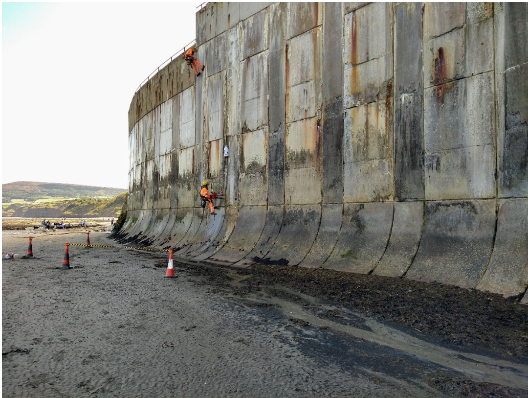
Photograph 1 – Seawall South end
