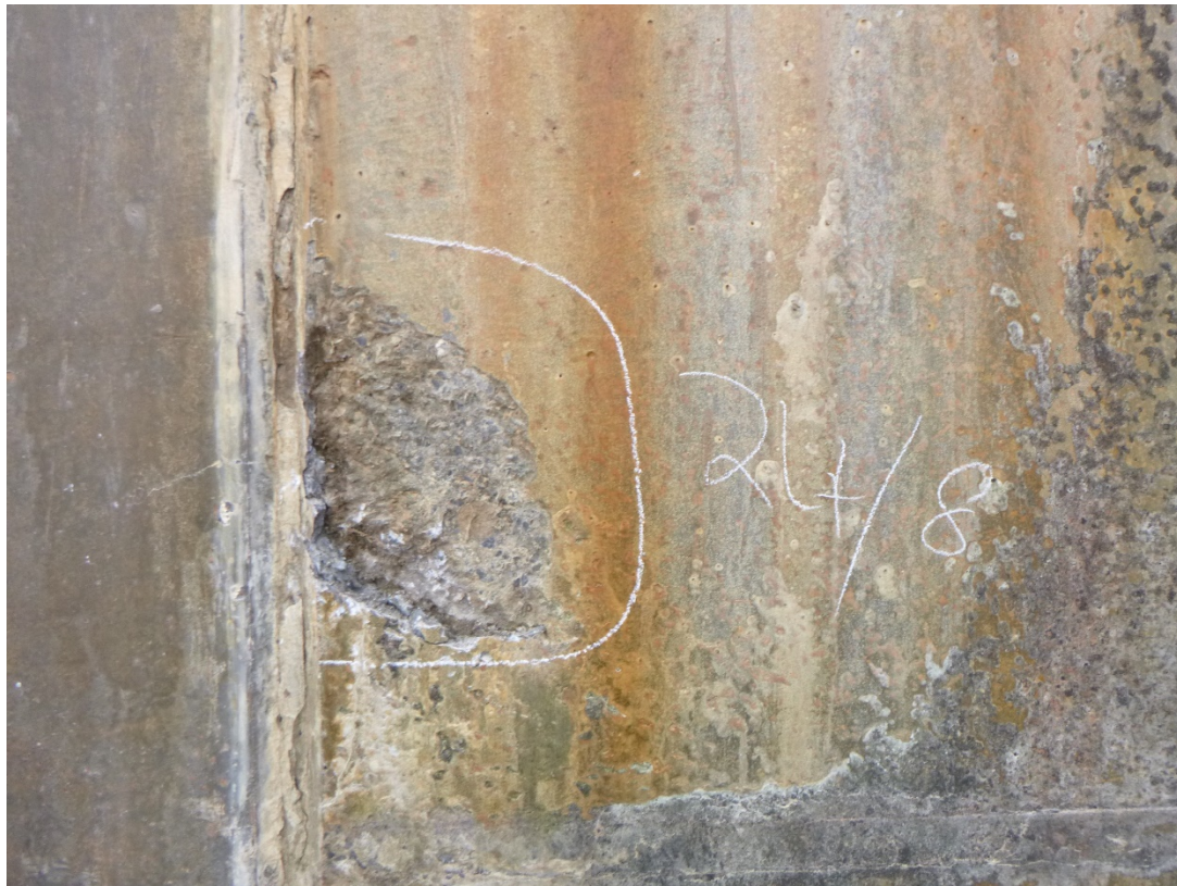
Photograph 7 – Defect 24-8 spalling
