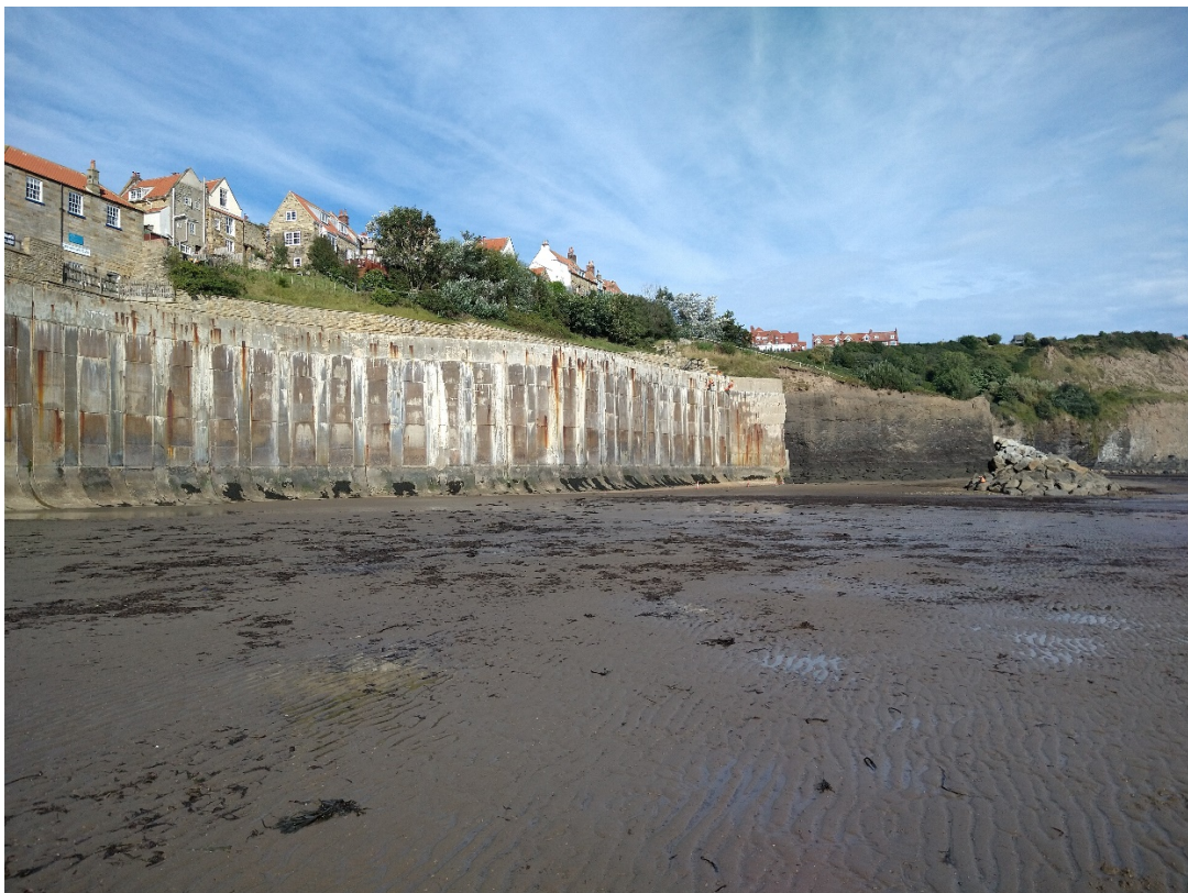
Photograph 2 – Seawall North end
